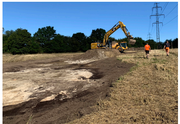
Figure 6. Construction of the lowland in september 2020. The nutrient-rich top soil is removed to expose the underlying nutrient-poor sandy soil which will encourage biodiverse vegetation.
